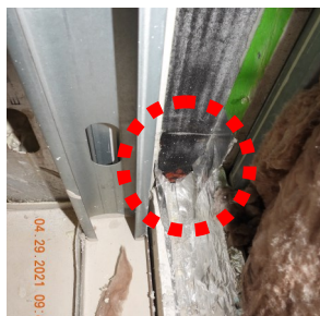
Int Floor & Ext Wall Joint — Different Manufacturers
